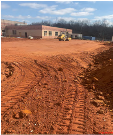
Grading building pad
