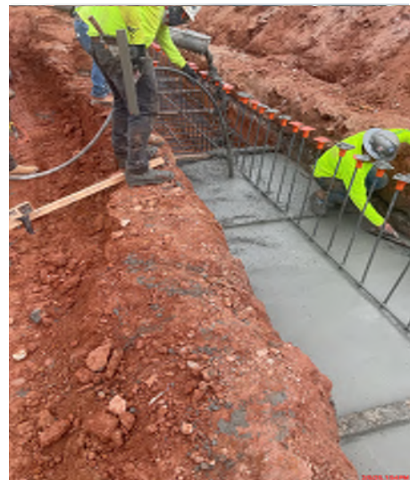
Pouring concrete in footing
