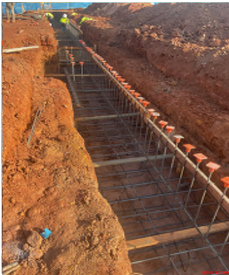
Installing and placing rebar and rebar mats in the footing
