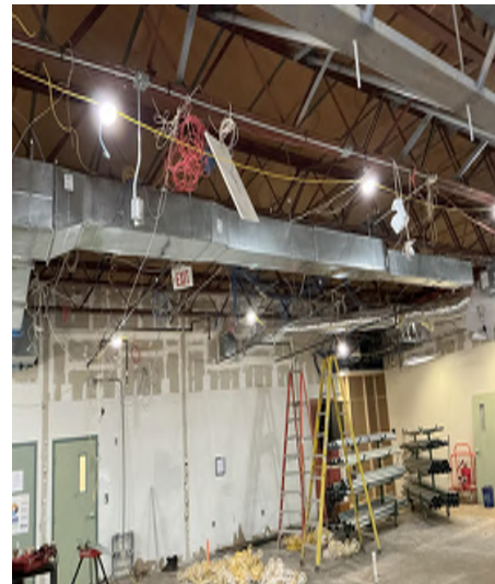
Ductwork installed in cafeteria
